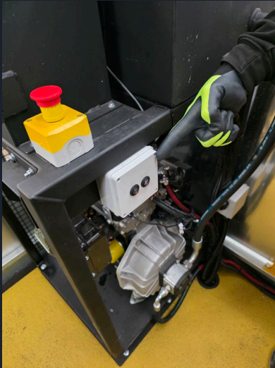
Left switch is Beacons
