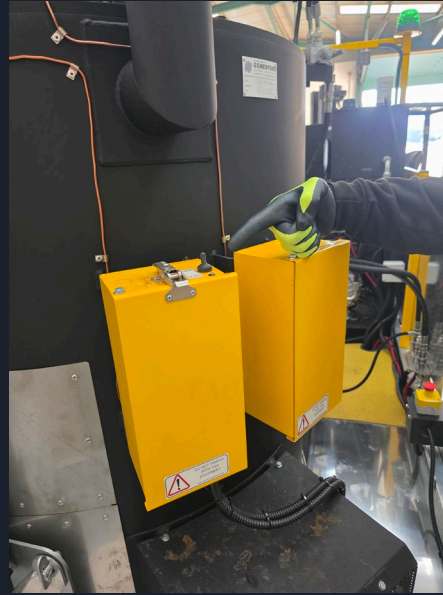
Burner ON switch
